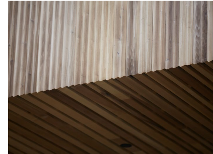
Thermally modified U.S. tulipwood cladding at Maggie’s Centre
