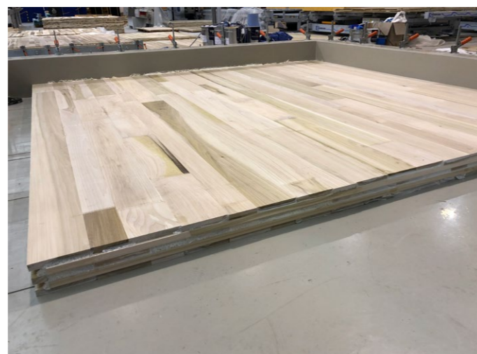
CLT panels in press after assembly time has elapsed
