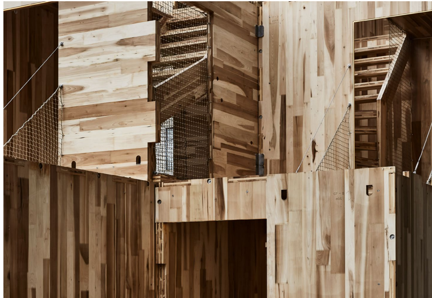
Tulipwood CLT panels of MultiPLY at its third iteration in Milan 2019
